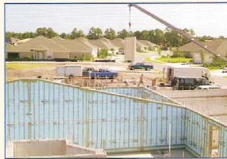
One of several residential developments built using EBS forms. These 200 homes were built at a rate of 4 structures per week.
